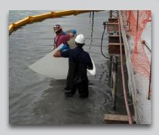
Transport the PileMedic™ sheet into water
