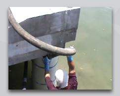
Mix grout and fill the annular space between the jacket and the pile with grout
