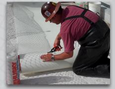
Cut PileMedic™ sheet to desired size
